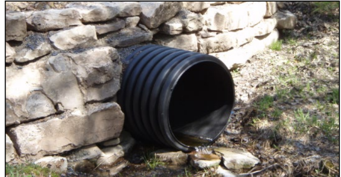
Stable stacked stone endwall
