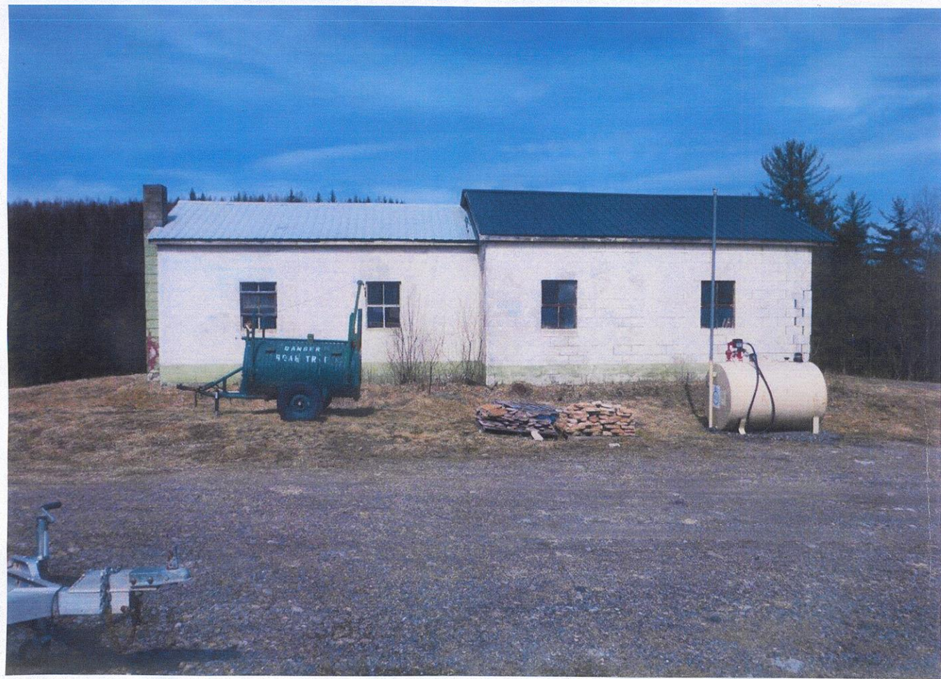
PICTURE OF BUILDING (SOUTH SIDE)
