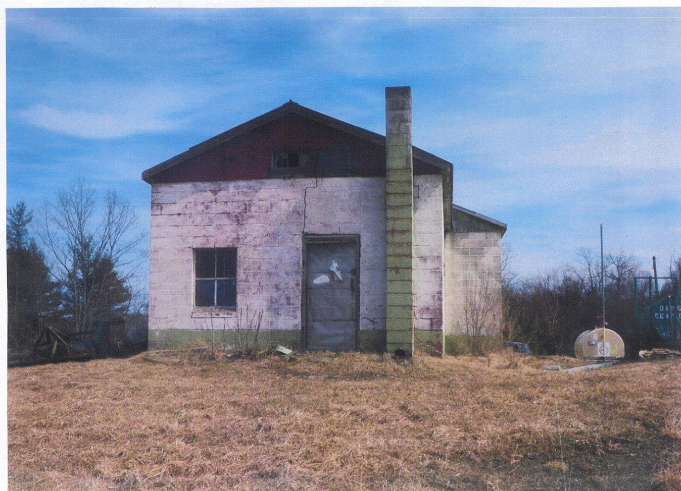
PICTURE OF BUILDING (WEST SIDE)
