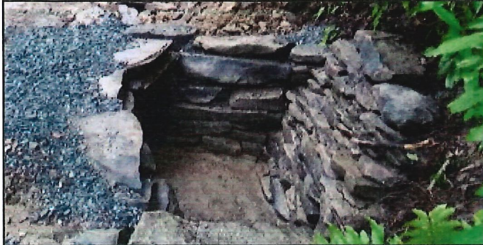
Stable headwall with bankwall
