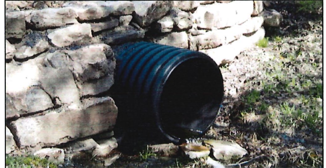
Stable stacked stone endwall
