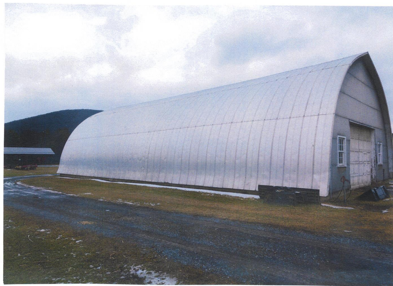
PICTURE OF BUILDING (WEST SIDE)
