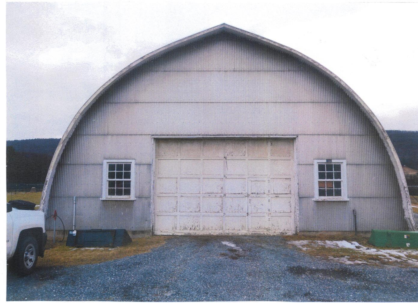
PICTURE OF BUILDING (SOUTH SIDE)
