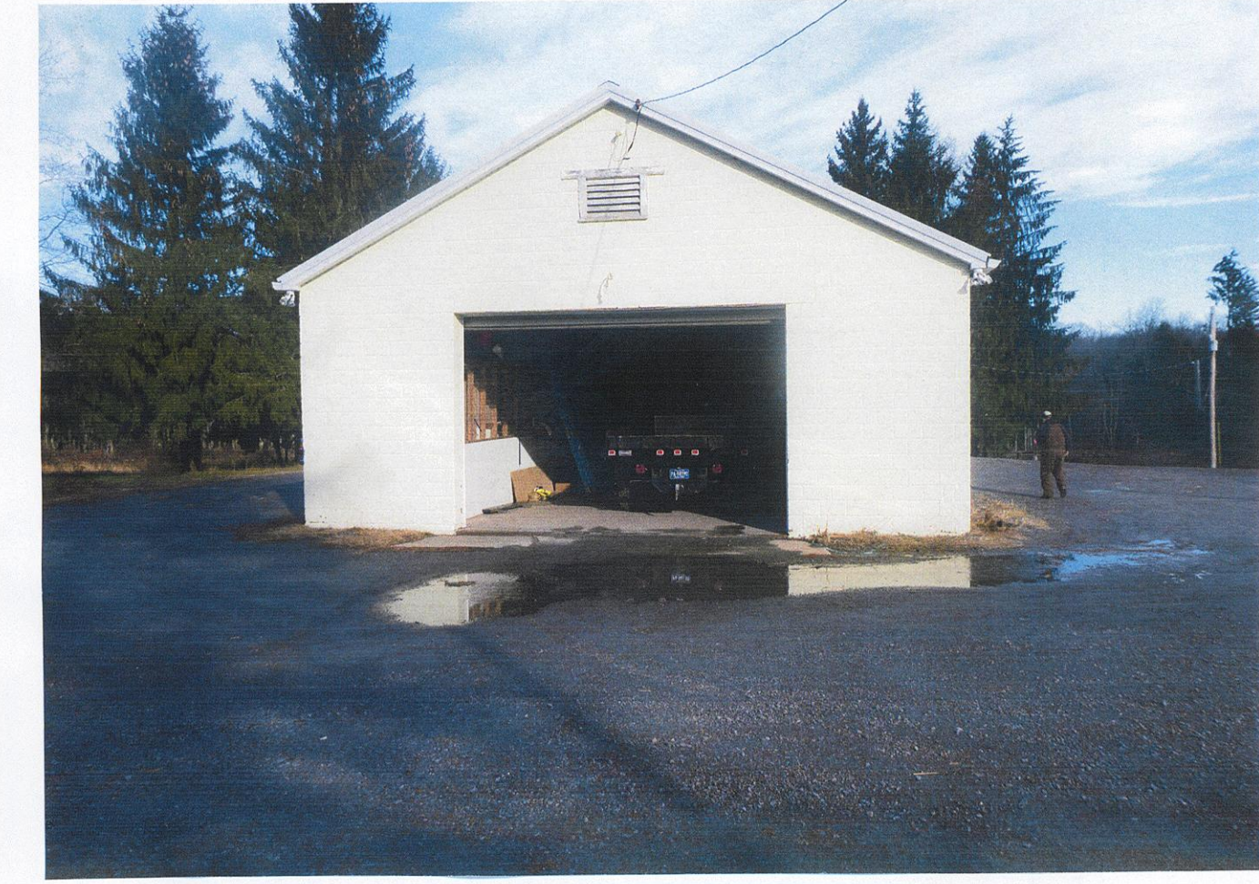
PICTURE OF BUILDING (SOUTH SIDE)
