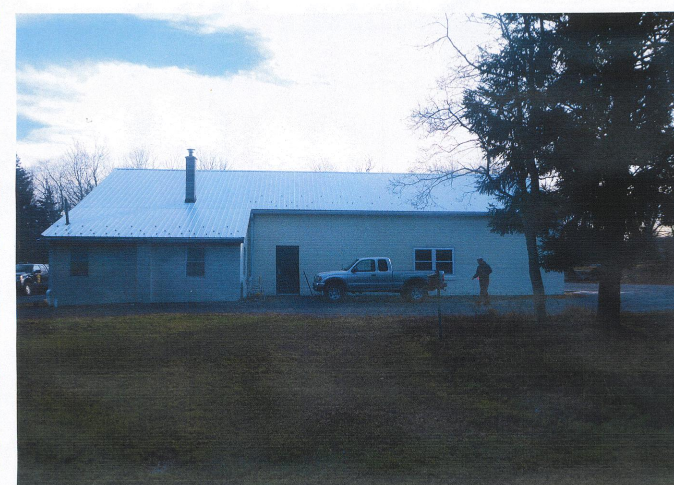
PICTURE OF BUILDING (WEST SIDE)
