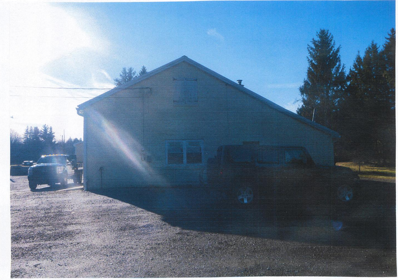
PICTURE OF BUILDING (NORTH SIDE)
