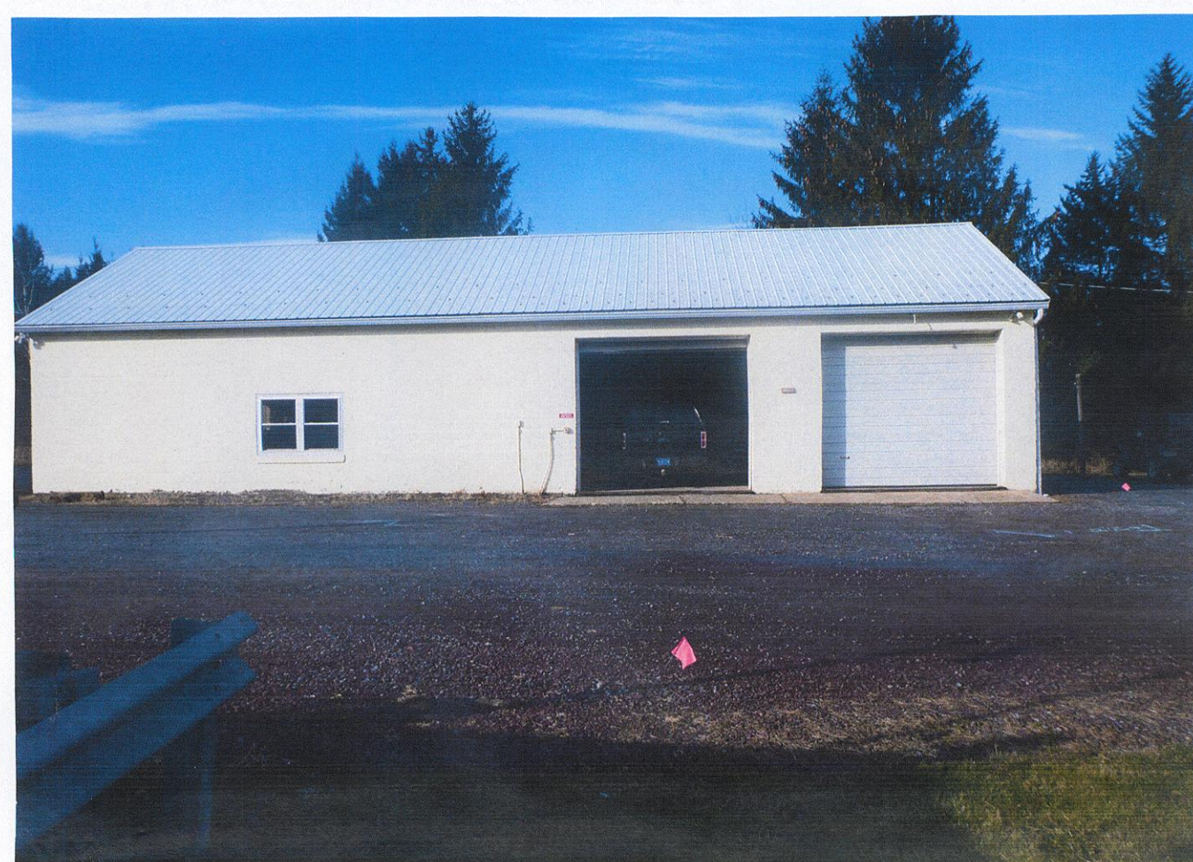
PICTURE OF BUILDING (EAST SIDE)
