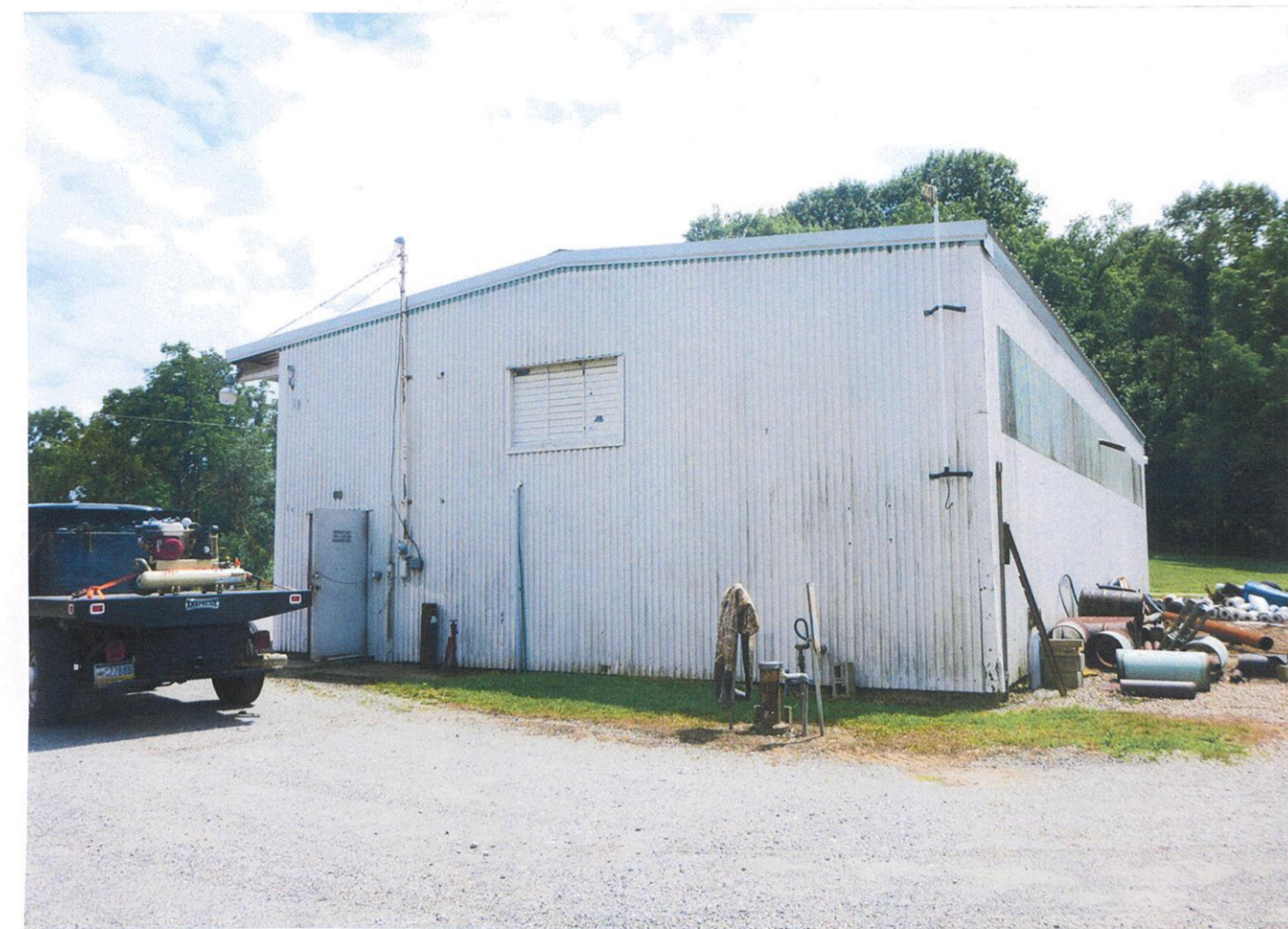
PICTURE OF BUILDING (NORTH SIDE)
