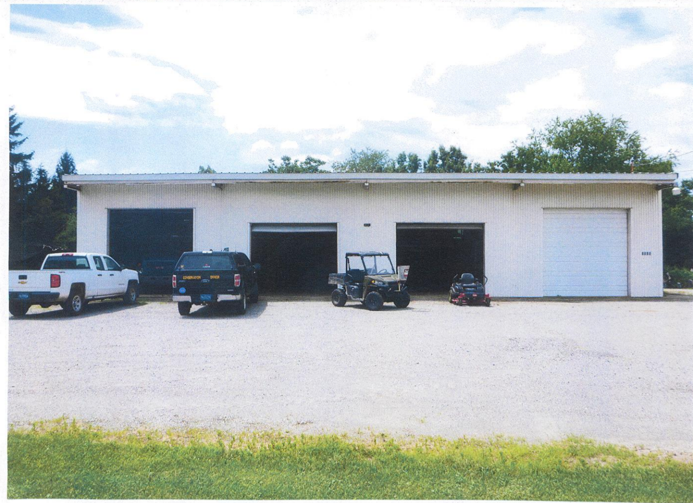
PICTURE OF BUILDING (EAST SIDE)
