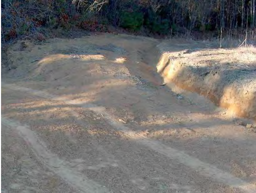
FIGURE 3.3 Typical Turnout
