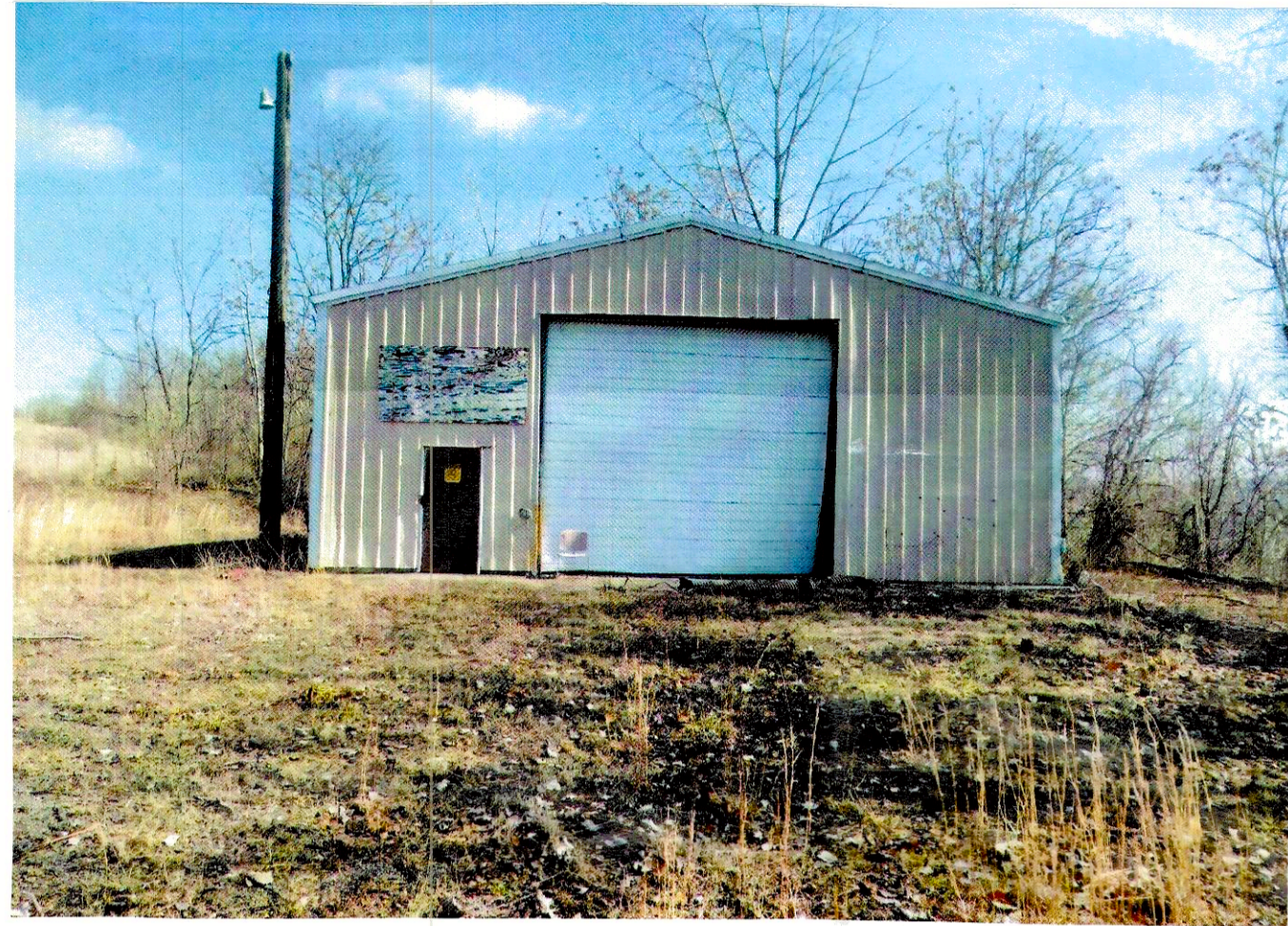
PICTURE OF STORAGE BUILDING (WEST SIDE)
