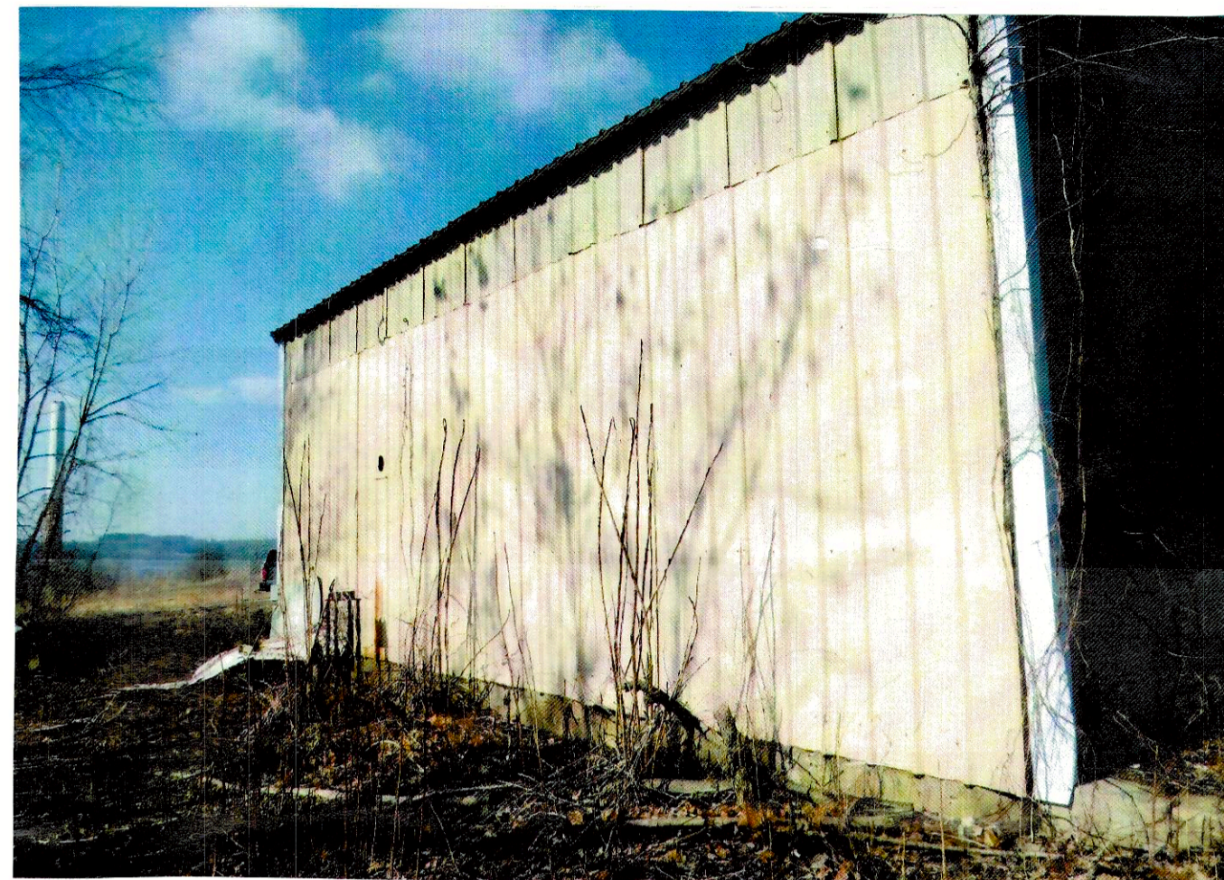
PICTURE OF STORAGE BUILDING (SOUTH SIDE)
