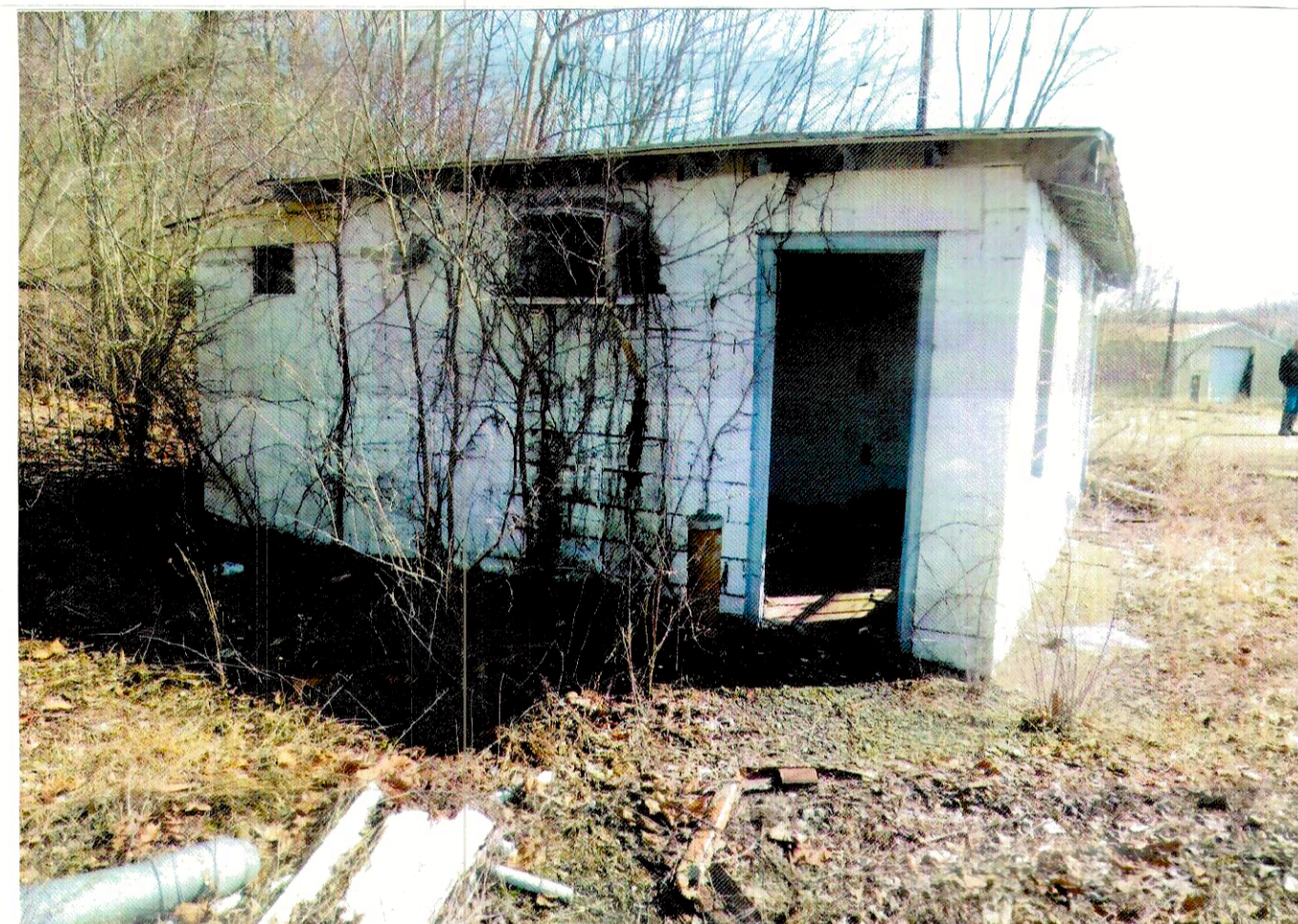
PICTURE OF SCALE HOUSE (WEST SIDE)
