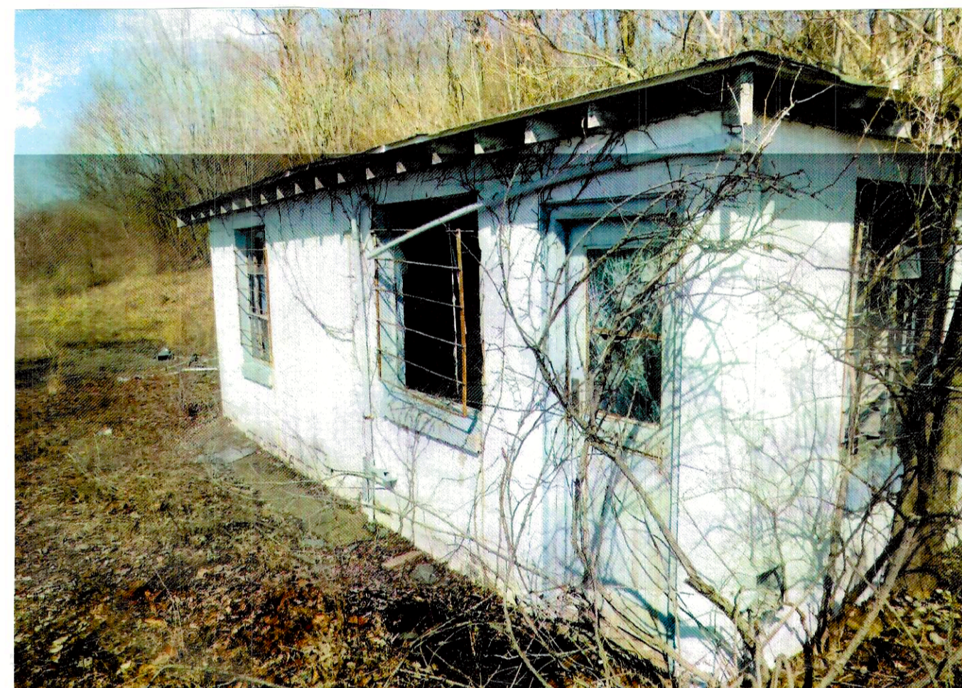
PICTURE OF SCALE HOUSE (SOUTH SIDE)
